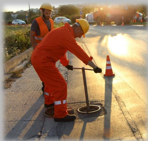
Checking the Low Pressure valves
