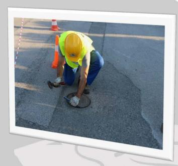
The Operational On-Call Technician, having notified the On-Call Officer of the incident and obtained approval, instructs the technician to shut off the valve 24-16 for the safe interruption of gas supply in part of the pipeline, in order to restore the damage.
