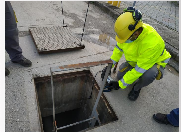
Shutting-off of the Medium-pressure Network valve
