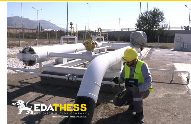
Leakage check at the entry point of the Northern Larissa distribution network.
